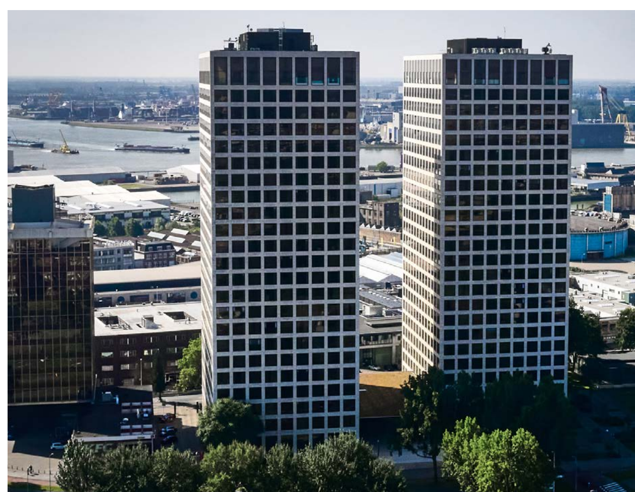
Lee Towers, Rotterdam
